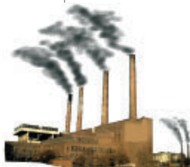
Factories to make fuel trucks
